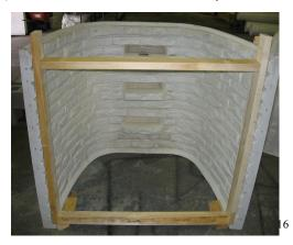
side to the concrete wall, then using  $4 \times 4$  posts and ratchet straps to pull well into proper width. Make sure the vertical post on free side is set back from flanges to allow access to mounting holes.
