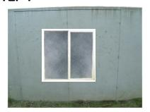
Locate finished grade line or desired height of window well and snap horizontal level chalk line.
